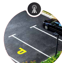
Sensor detecting occupied parking slots
